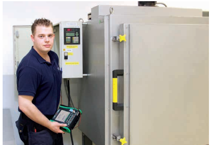
Maintenance Technician at work ( CQI-9 or AMS 2750 E )
